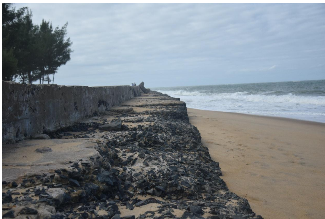
Figure 30: Digue de protection
