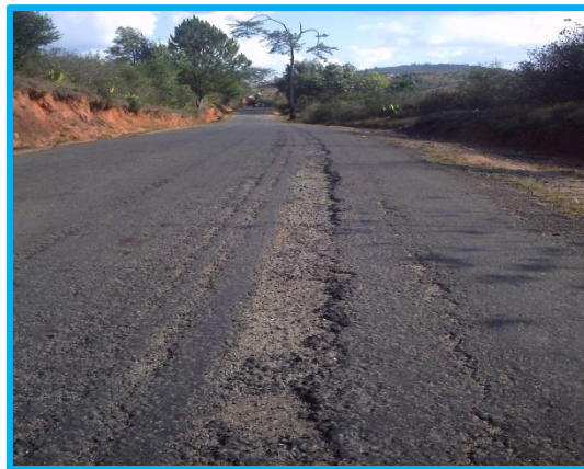
Figure n°4 Ravinement longitudinal
