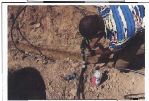
Installation de Vannes
