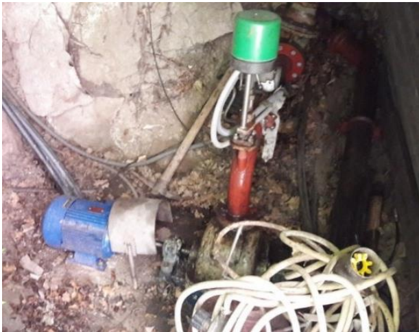
Figure 35: Turbogroupe 4 (4 kW)
