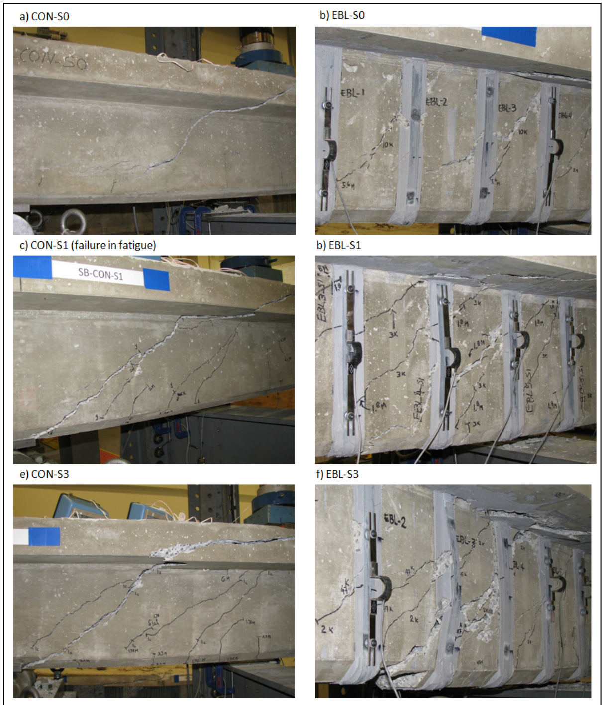
Figure 5.4 Crack patterns at failure of test specimens
