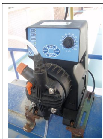
Figure n°11: Machine doseuse
