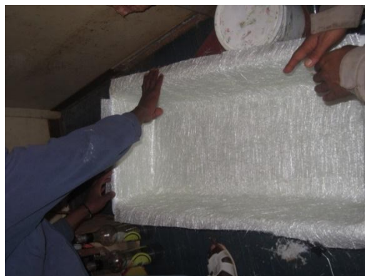
Figure 34: pose des mats 300g/m 2
