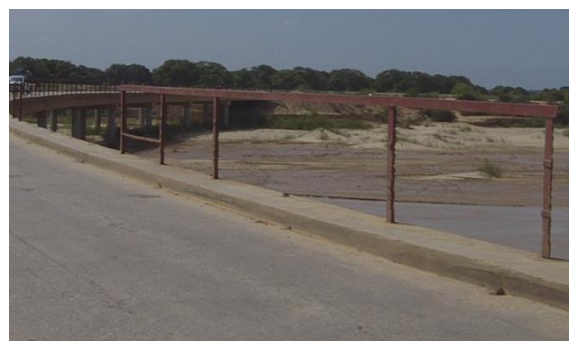
Photo 11 Insuffisance de garde-corps
