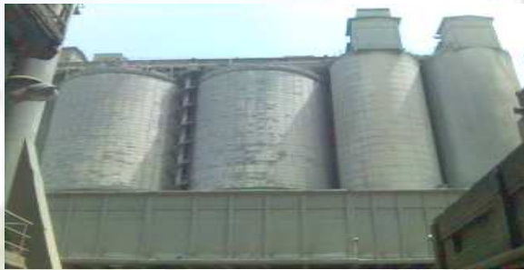
Figure 11: Stockage du ciment
