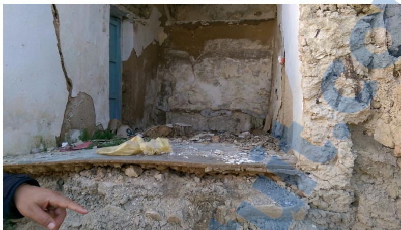
Figure 55 . construction sans fondations
