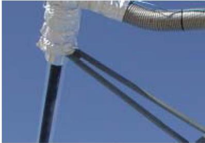
Figure 2. 5: le support de tube absorbeur [76]
