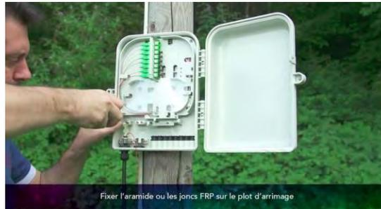
**FIGURE 50: POINTS DE BRANCHEMENT OPTIQUE AVEC CONNECTEURS**
