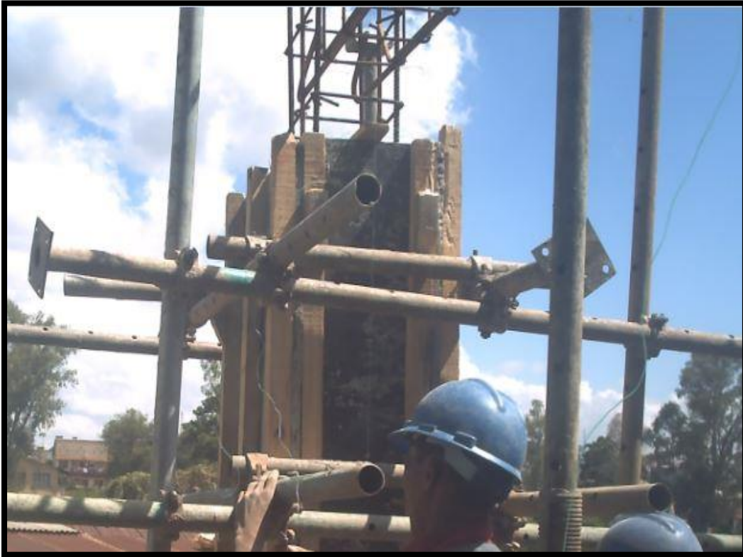
Figure 40: Coffrage du poteau
