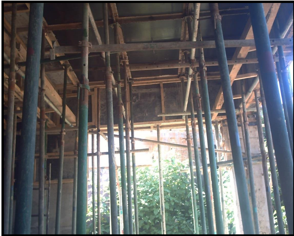
Figure 42: Coffrage de la dalle
