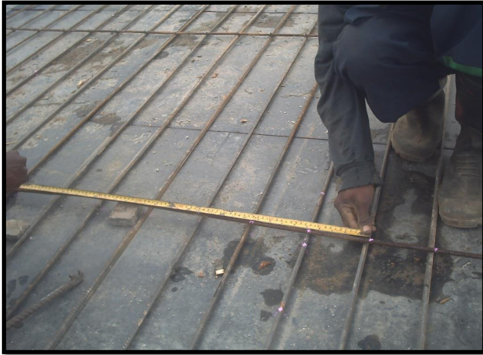
Figure 43: Ferraillage de la dalle
