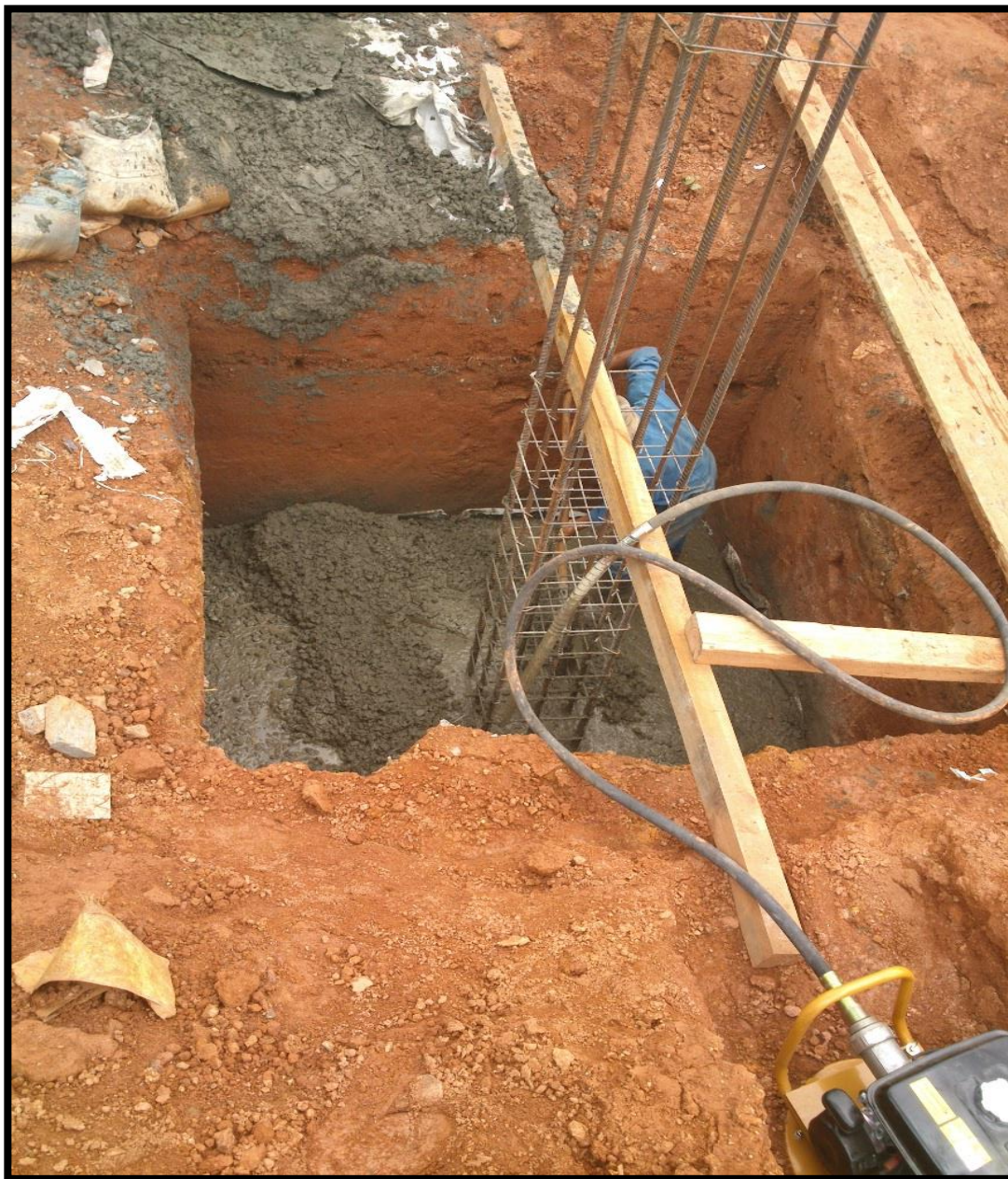
Figure 38: Coulage de beton
