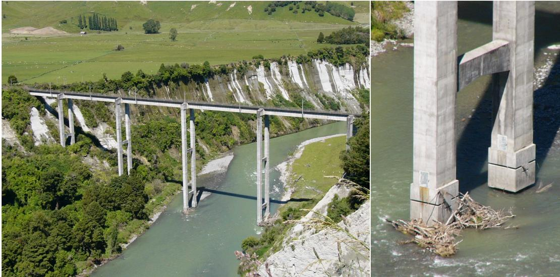
**Figure 1-2 – a) The South Rangitikei Viaduct, b) a close up of rocking hinge at the pier base**
