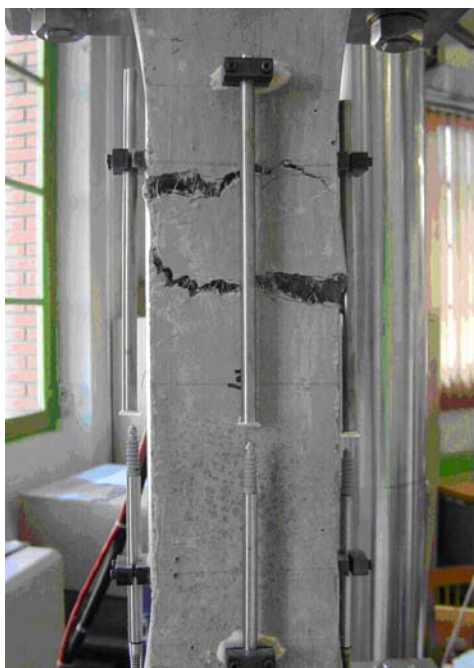
Figure 1.21. Multi fissuration du CEMTEC® en traction directe.
