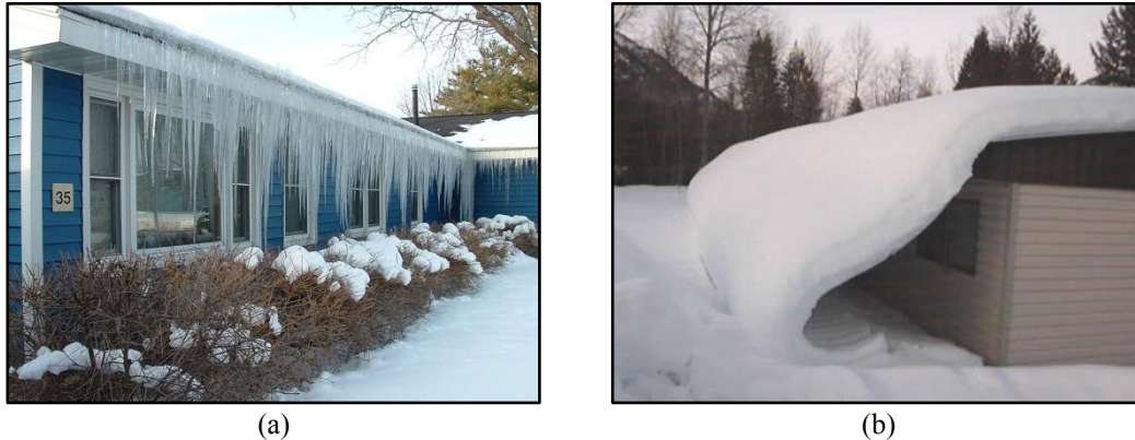
Figure 3. (a) An example of icicles formation on a building [9]. (b) A snow sliding phenomenon [10]
