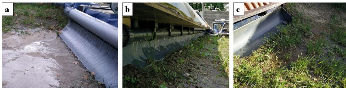
Figure 0.5 (Figure S4). Runoff simulator and surface runoff drainage system. a The runoff simulator generated longitudinal inflows at the upstream end. b The runoff simulator generated lateral inflows along the swale channel. c The gutter drained non infiltrated flow at the downstream end (standard swale)
