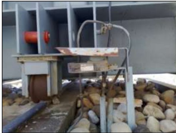
Figure III.10 : Protection Masse cuve
