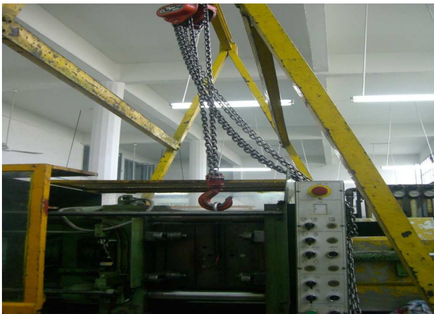
Figure 15: Manutention manuelle du moule suspendu
