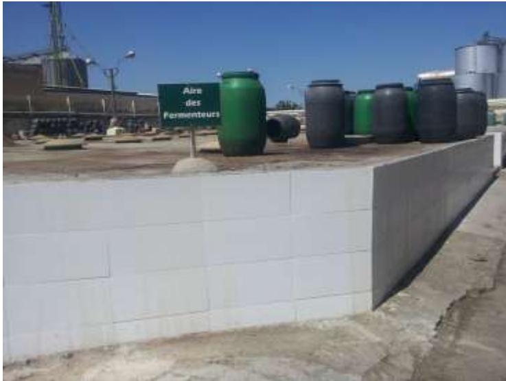
Figure 44: cuves de fermentation
