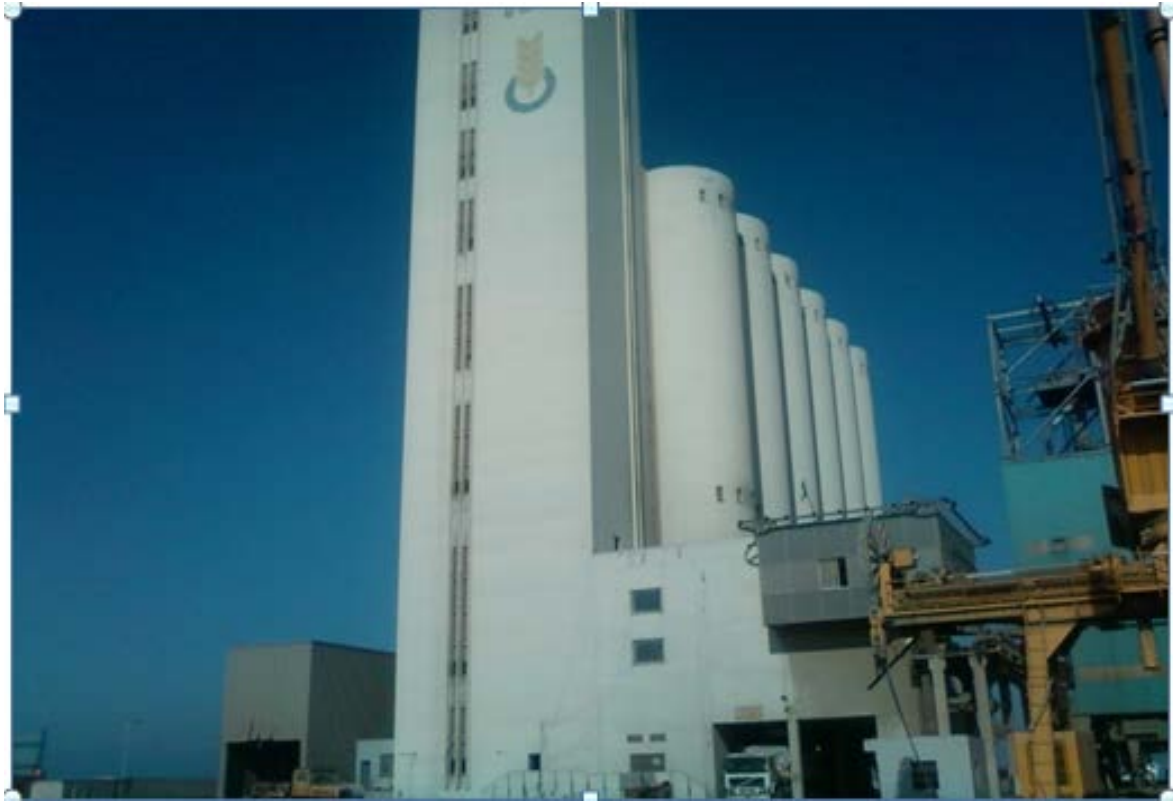
Photos n°05 : Complexe Ghazaouet (Tahraoui,2016).
