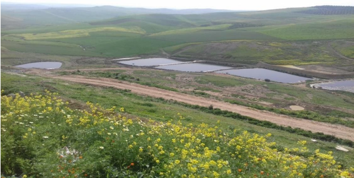
Figure 14: Bassins de lixiviat
