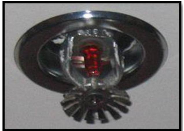
Figure 27: Splinkler
