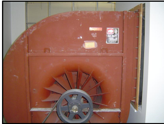
Figure 3.3 Double impeller centrifugal fan
