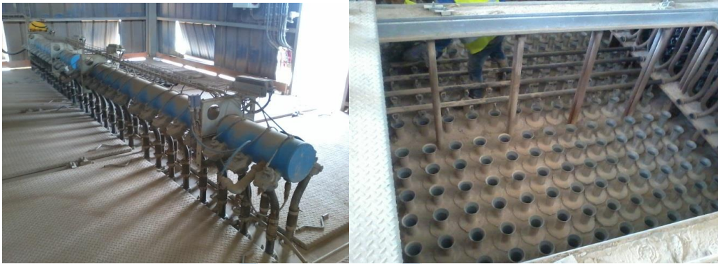
Figure 33: Filtre process charbon
