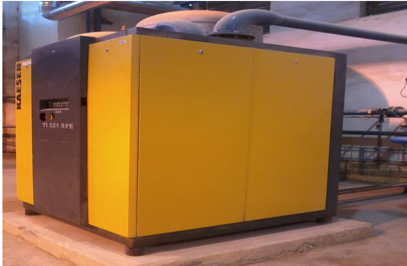
Figure 27: Le sécheur frigorifique
