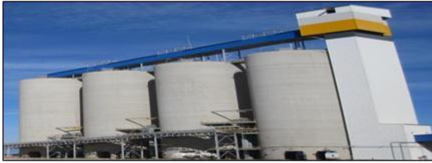
Figure 9: Silos de stockage du ciment
