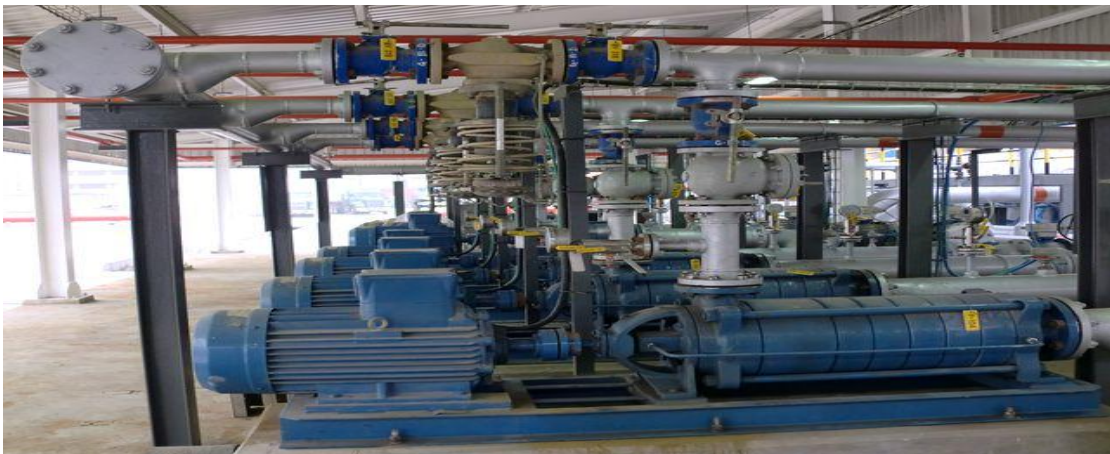
Figure 12 :les Pompes de GPL
