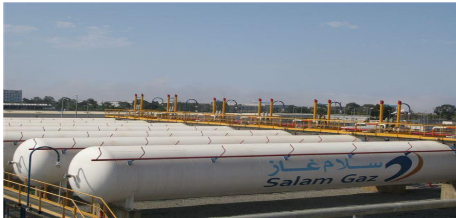
Figure 7 :Stockage de GPL
