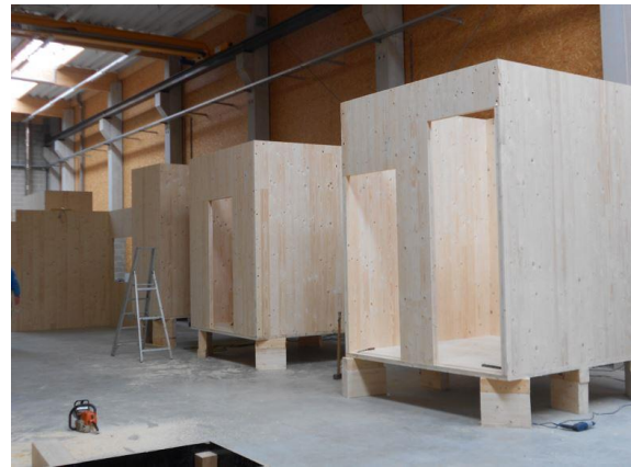
Figure 106 : Construction en atelier_Ncube_Naturhome.
