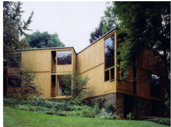
Figure 73 : Façade arrière_Fisher House [Cal21].
