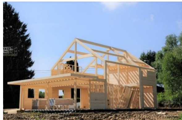
Figure 40 : Construction en poteaux-poutres [Sta21].
