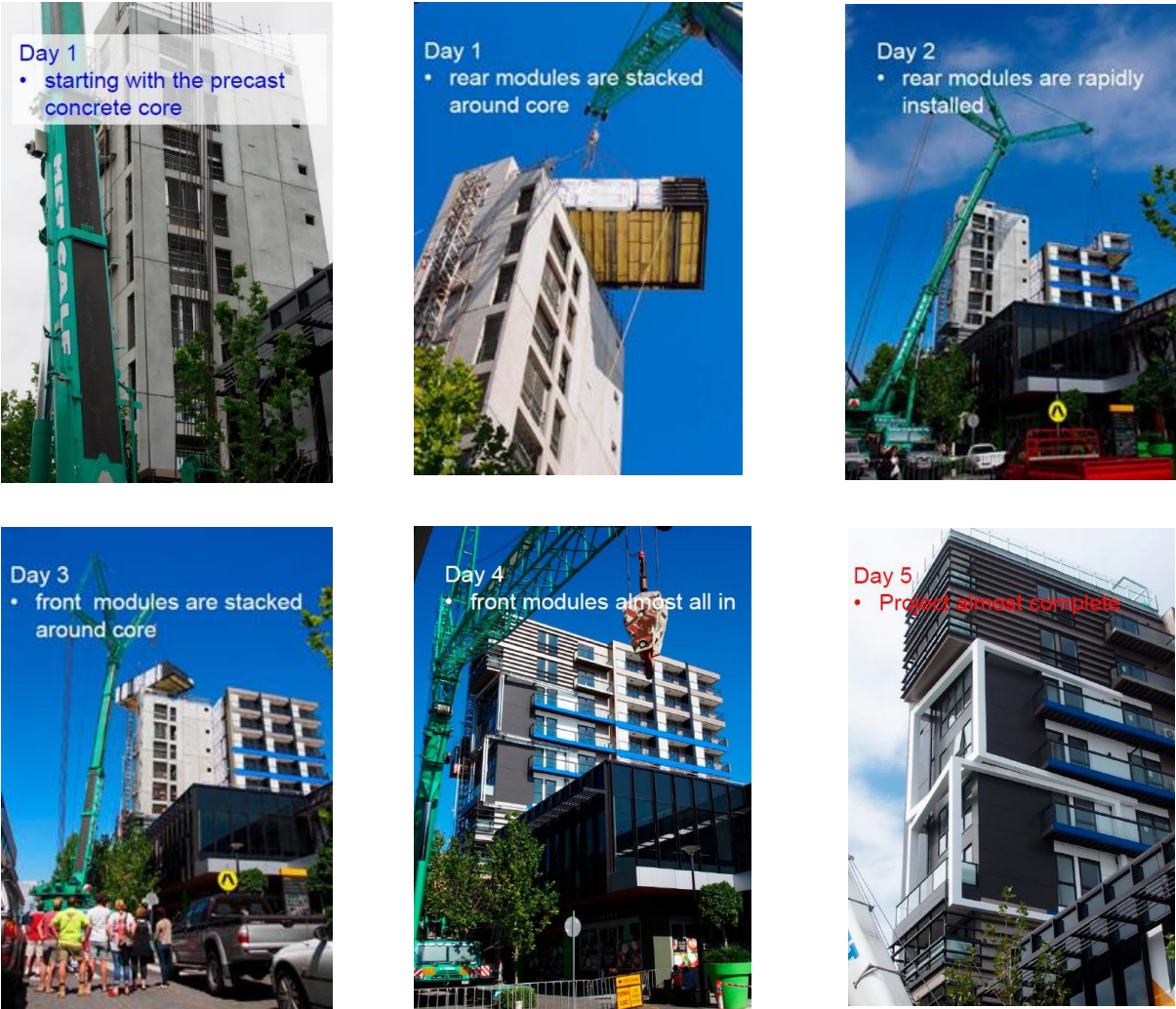
Figure 50 : One9 modular building stabilized by a concrete core [BKK16].
