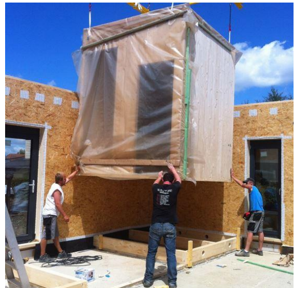
Figure 107 : Pose des modules 3D_Ncube_Naturhome.
