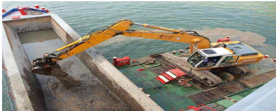
Figure 1.3 Dragage mécanique (BOUKEMMOUM N., NOUAOURIA A. (2019))
