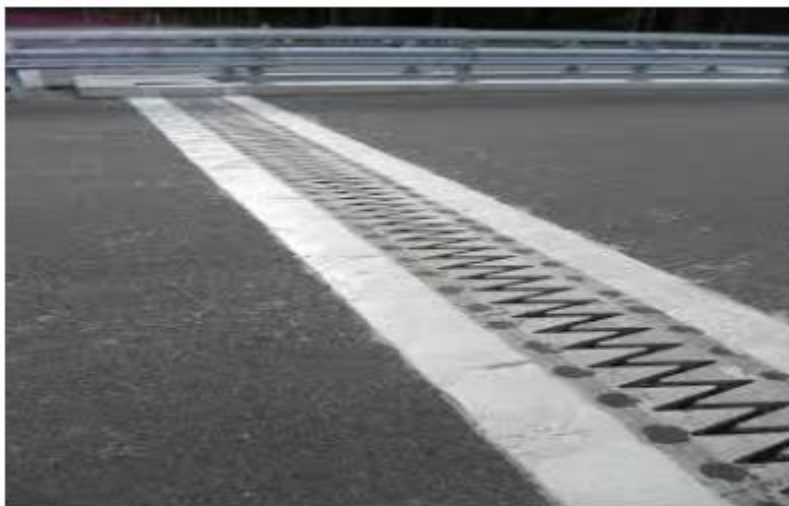
Figure 27:les joints de pose
