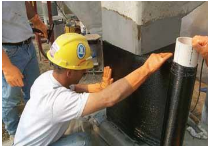
(a) Renforcement d'un poteau [3]
