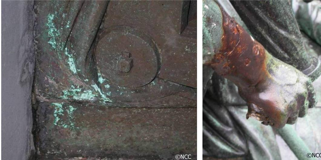
Figure 11 Left: Active corrosion on a bas-relief.
