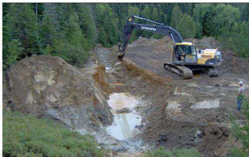
Figure 6.4 Excavation du drain DOL-3
