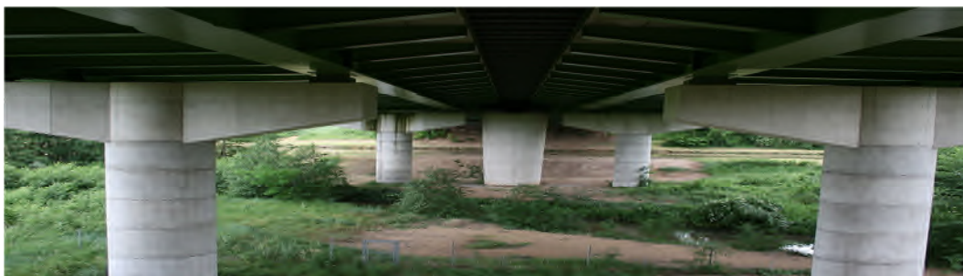
Figure I.10. Photo des piles marteaux [3]
