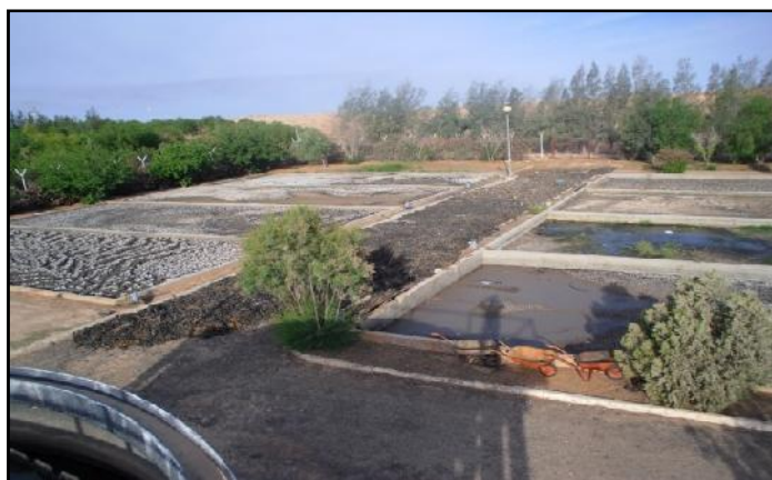
Figure III.14: Lit de séchage (22/05/2012)
