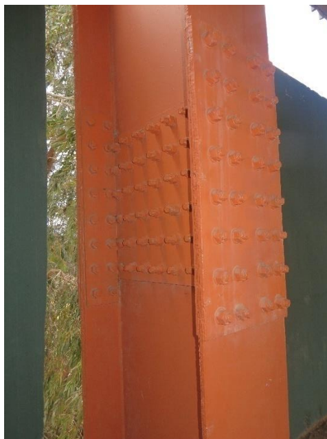
Figure II. 6: Assemblage poteau-poteau
