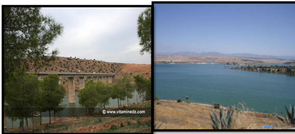
Figure 2.8: Barrage Hamam Boughrara (Khaladi A., 2008).
