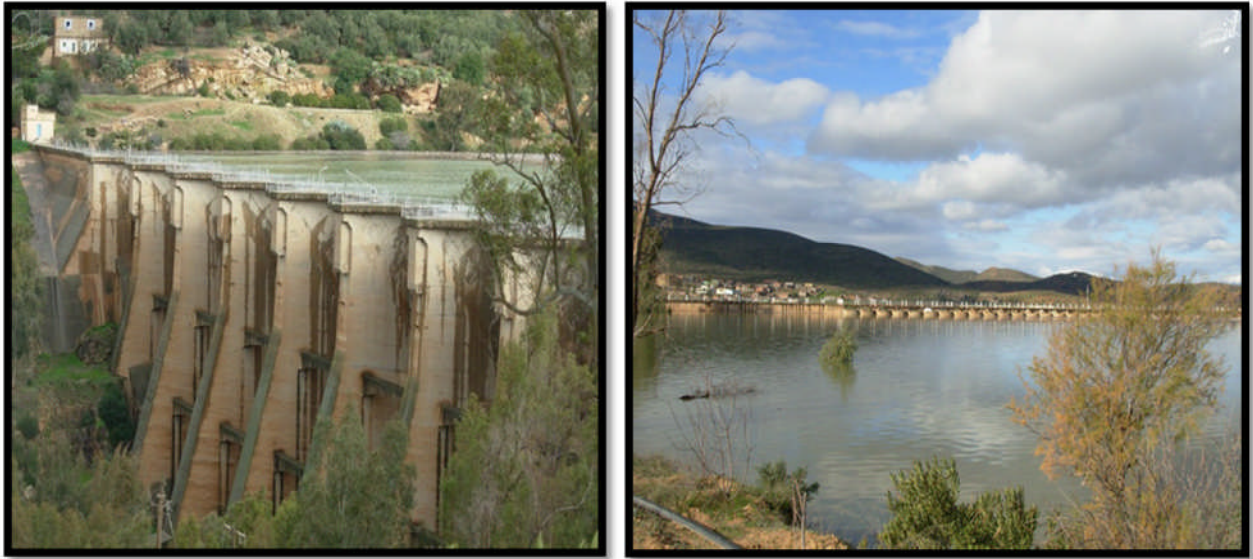
Figure 2.7: barrage Beni Bahdel (Photos Draou S., 2013).
