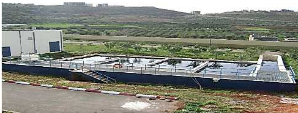
Figure III.10 : Bassins de chloration
