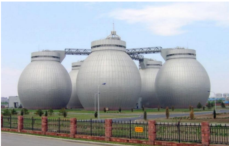
Figure I.15: digesteurs (Master's project on organic waste digestion , 2017)
