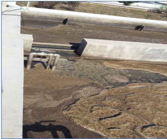
Figure III.15: Photo de la lame deversante retour de surnageant.
