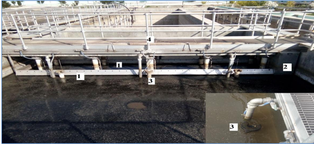
Figure III.13 : Photo de clarificateur ClarActor.
