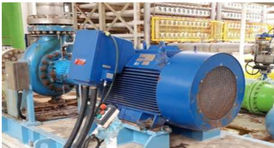
Figure III. 10 : Pompe booster.
