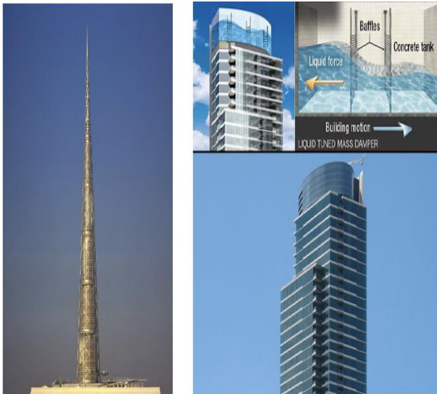
Photo 2.8 Systèmes TLDs a) millennium tower-Tokyo b) one rinconhill-San francisco [6].
