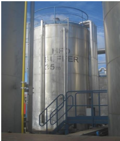
Figure 13 : Fuel buffer tank(HFO)
