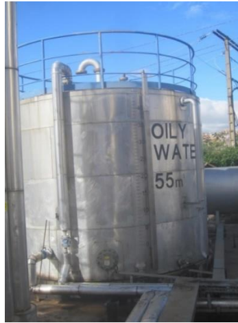
Figure 17 : Photographie Oily water tank
