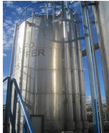
Figure 13 : Fuel buffer tank(HFO)
