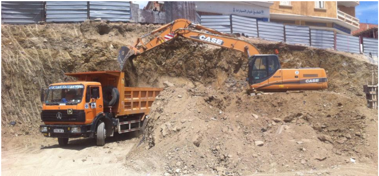
Figure 28: Excavation en masse.
