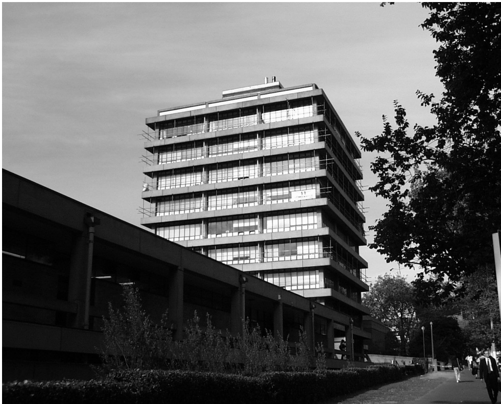
Figure 3.6: External view of the Engineering School Tower.
