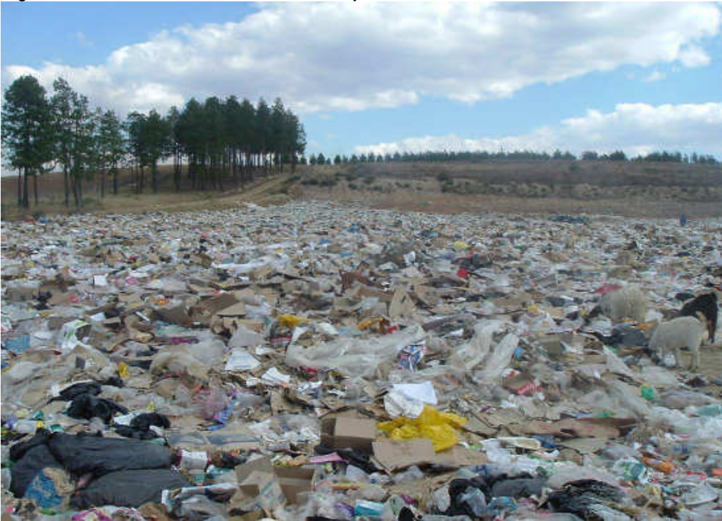
Figure 2-4. The same landfill site a year later. Note the lack of covering of the waste, the presence of goats on site and the partial removal of the tree screen.
