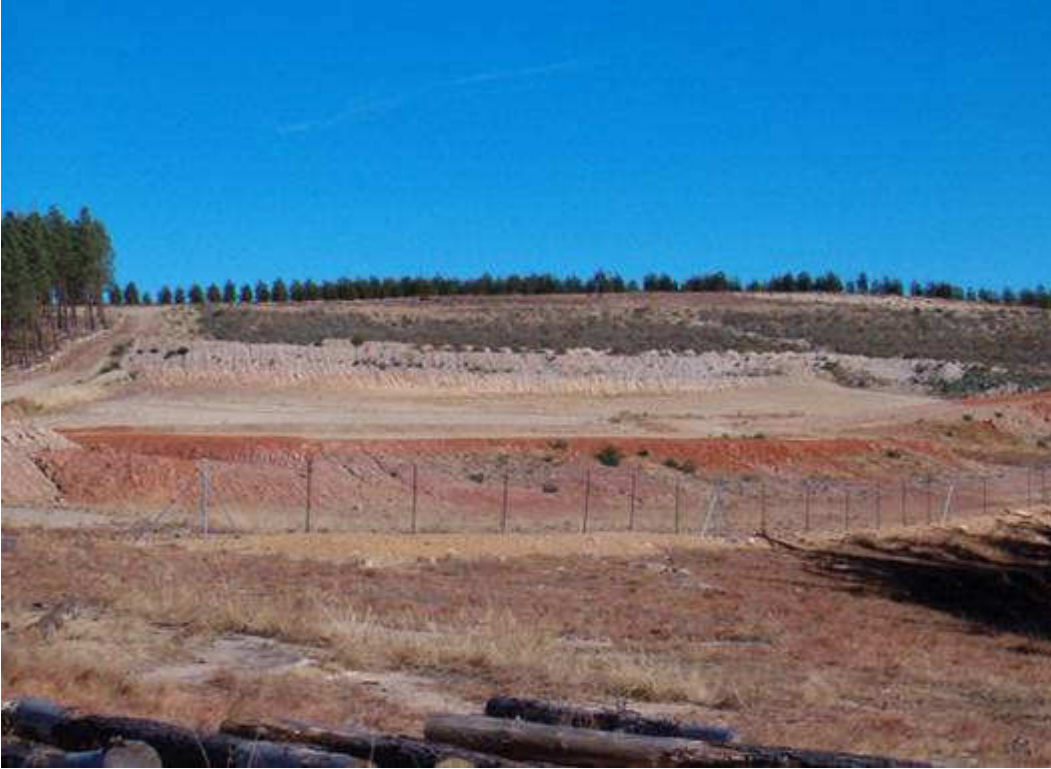
Figure 2-3. Landfill site in the Elundini area just after construction.
