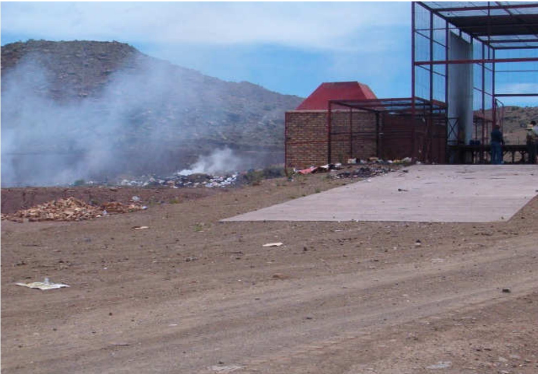
Figure 4-3. The incinerator that was installed at a landfill site in the Maletswai area in 2003 and was not operational at the time of follow-up a year later (note missing chimney). Waste was instead being burned on site.
