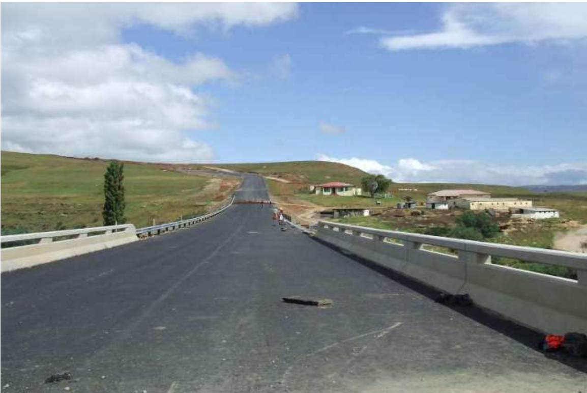
Figure 3-2. The same road and bridge after completion of the bulk earthworks but before all rehabilitation had been carried out.
