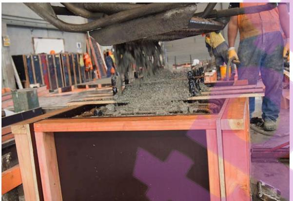
(b) Casting of concrete into foundation block
