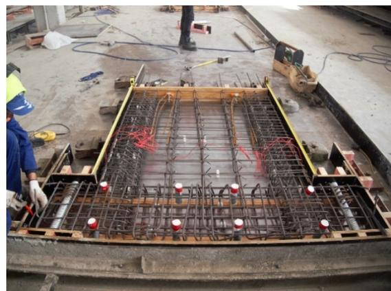
b) As-built detailing of wall M7
