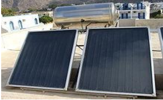
Figure 1.2: Solar Thermal Collectors: Flat plate collector and Evacuated tube [1.18]
