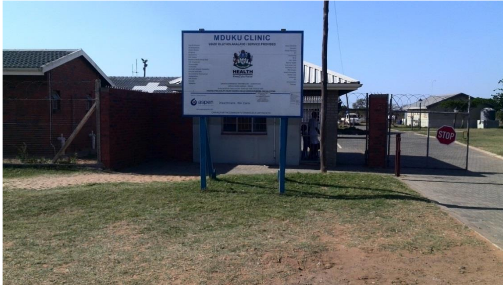
Figure 3.3: Mduku Clinic (A milestone project servicing more than 33000 people, unlike the mobile clinics with poor health services which used to exist) [Photograph by J.M. Muzirambi, 2016]
