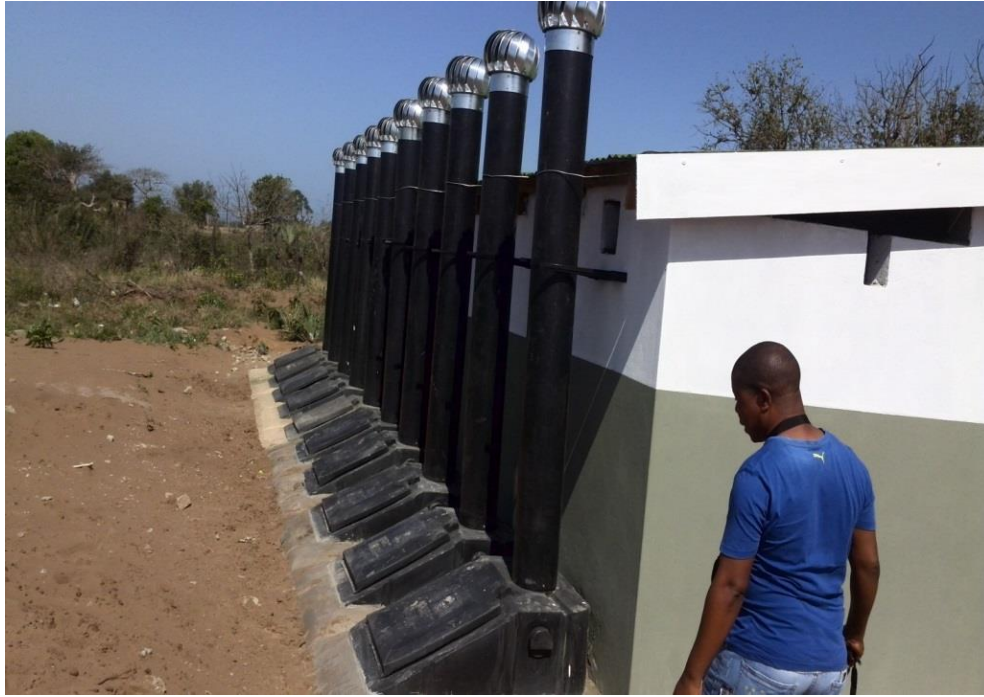
Figure 3.6: Modern biodigester toilet block at Nkomo Primary School, Mngobokazi (Improved health for the children) [Photograph by J.M. Muzirambi, 2016]
