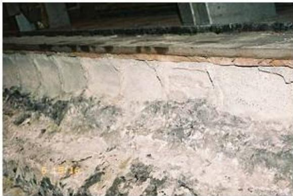
*Figure 3-2: Degradation of SNBSC at the upper level of the sideling [35].*
