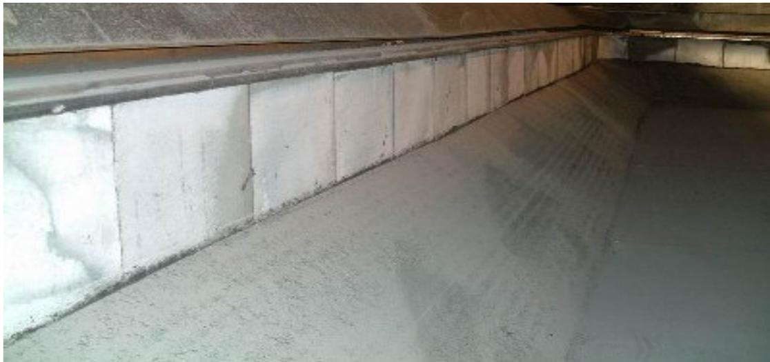
*Figure 1-6: Picture taken from reduction cell, the sidewall with SNBSC bricks at the top and ramming paste slope at the bottom above the cathode surface.*
